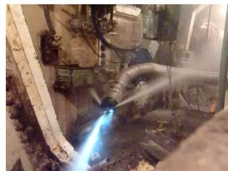
Fig 5 JetSnake water jetting – inside TBM
