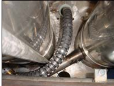
A snake-arm robot in the Ringhals nuclear power plant
