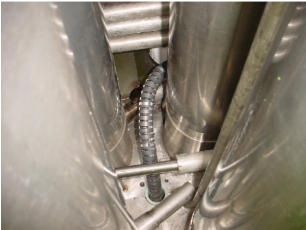
Figure 3 - Underneath arm snaking into position
