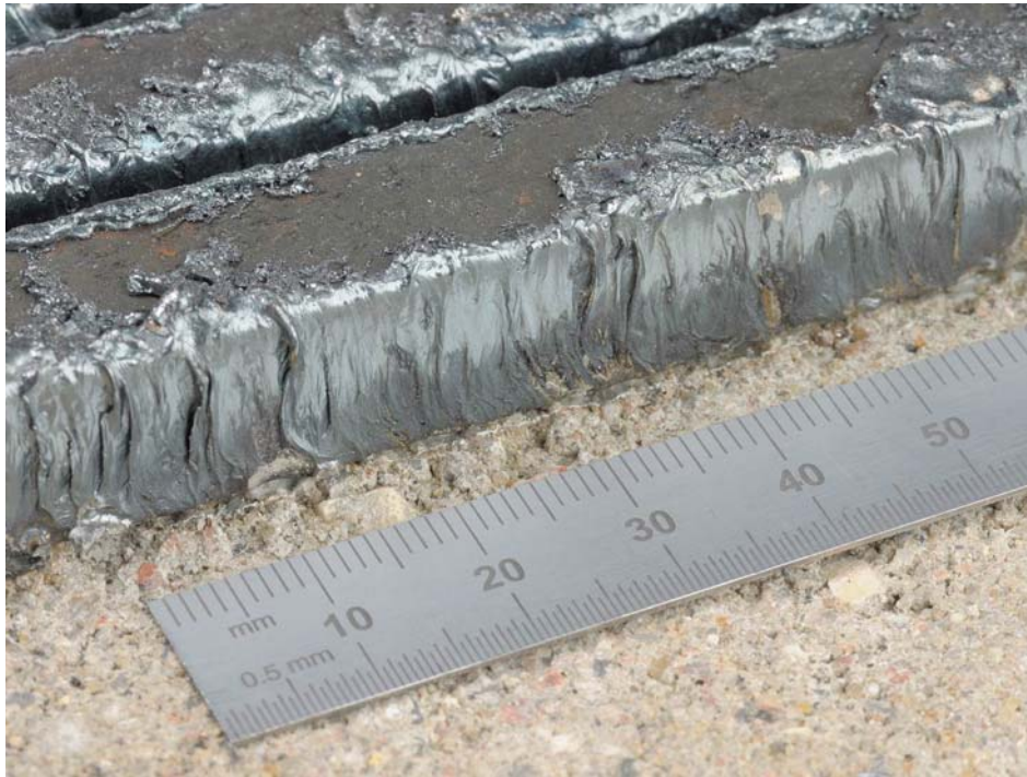
Figure 11 Gouge cutting of 12mm thick CMn steel on top of concrete, with minimum damage to the concrete surface.
