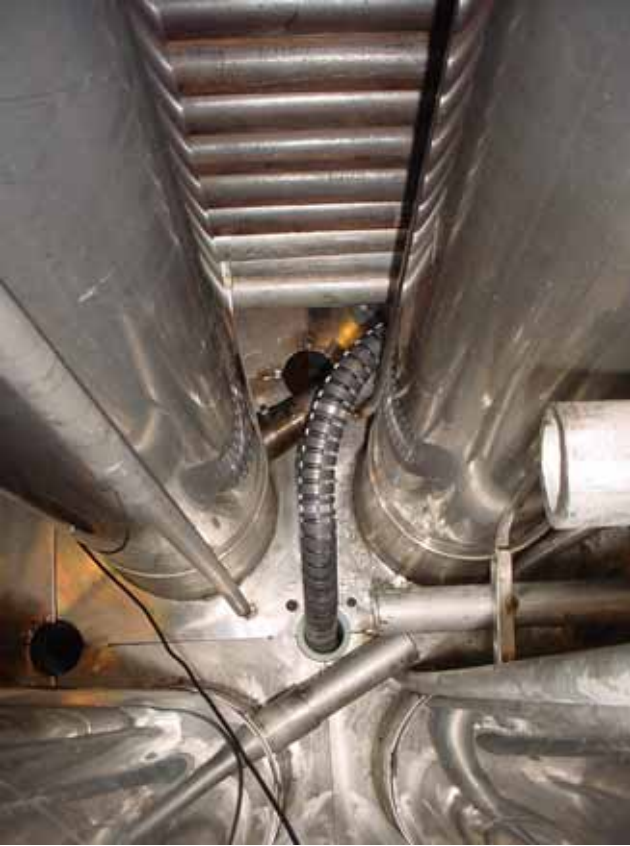
Figure 10 - UA in position
