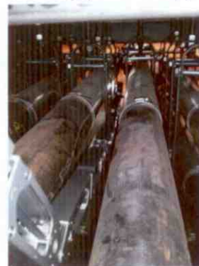
Figure V.5: OPG arm deployed below the walkway (in mock-up)
